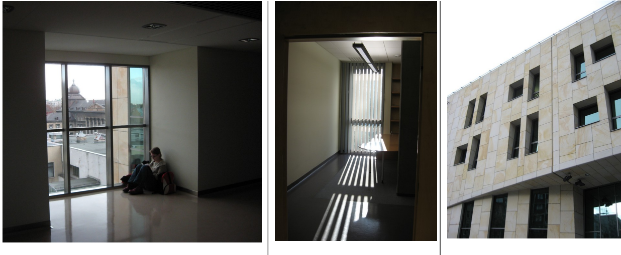
Figure 1,2,3. Faculty of Theology. University of Silesia - recess by the window and a big glazed surface enabling an interesting view on the city - constitute a place for relaxation; unfavourable patterned shades cast by vertical blinds; deeply mounted windows of the southern facade preventing the overheating of the interior space (photo Joanna Tymkiewicz).
