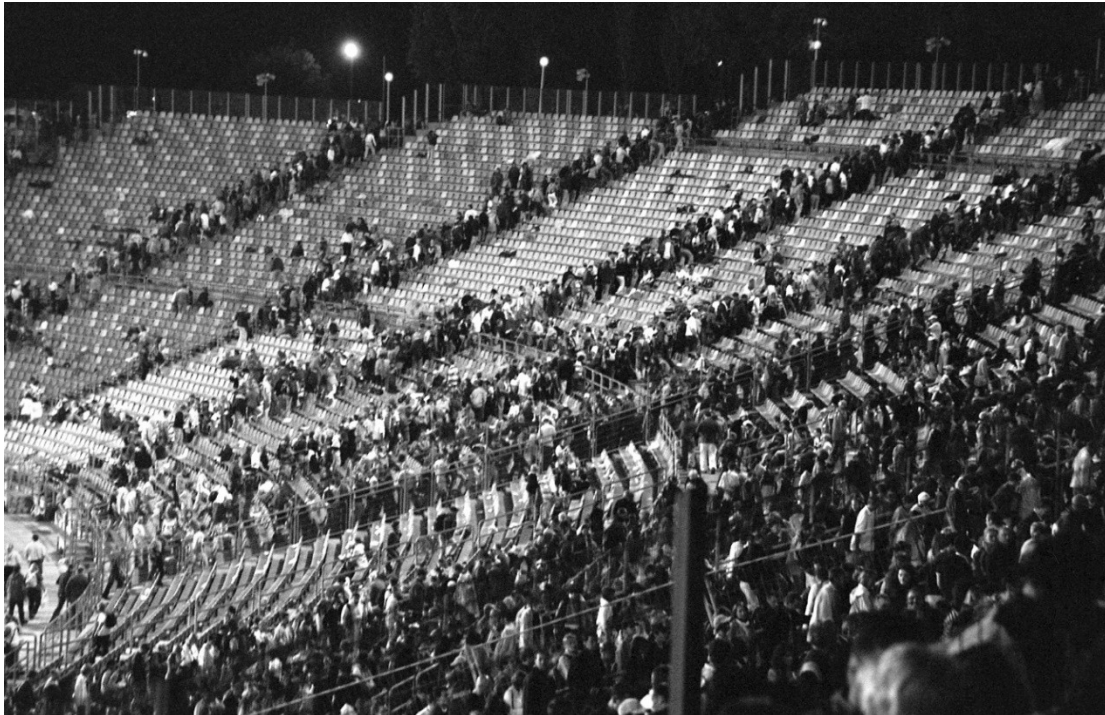
Figure 6. The Silesian Stadion, Chorzow, Poland - moment of leaving the stands by the audience after the concert. Evacuation routes parameters allow to reach evacuation time shorter than 5 minutes. (Photo: Z. Pelczarski)
