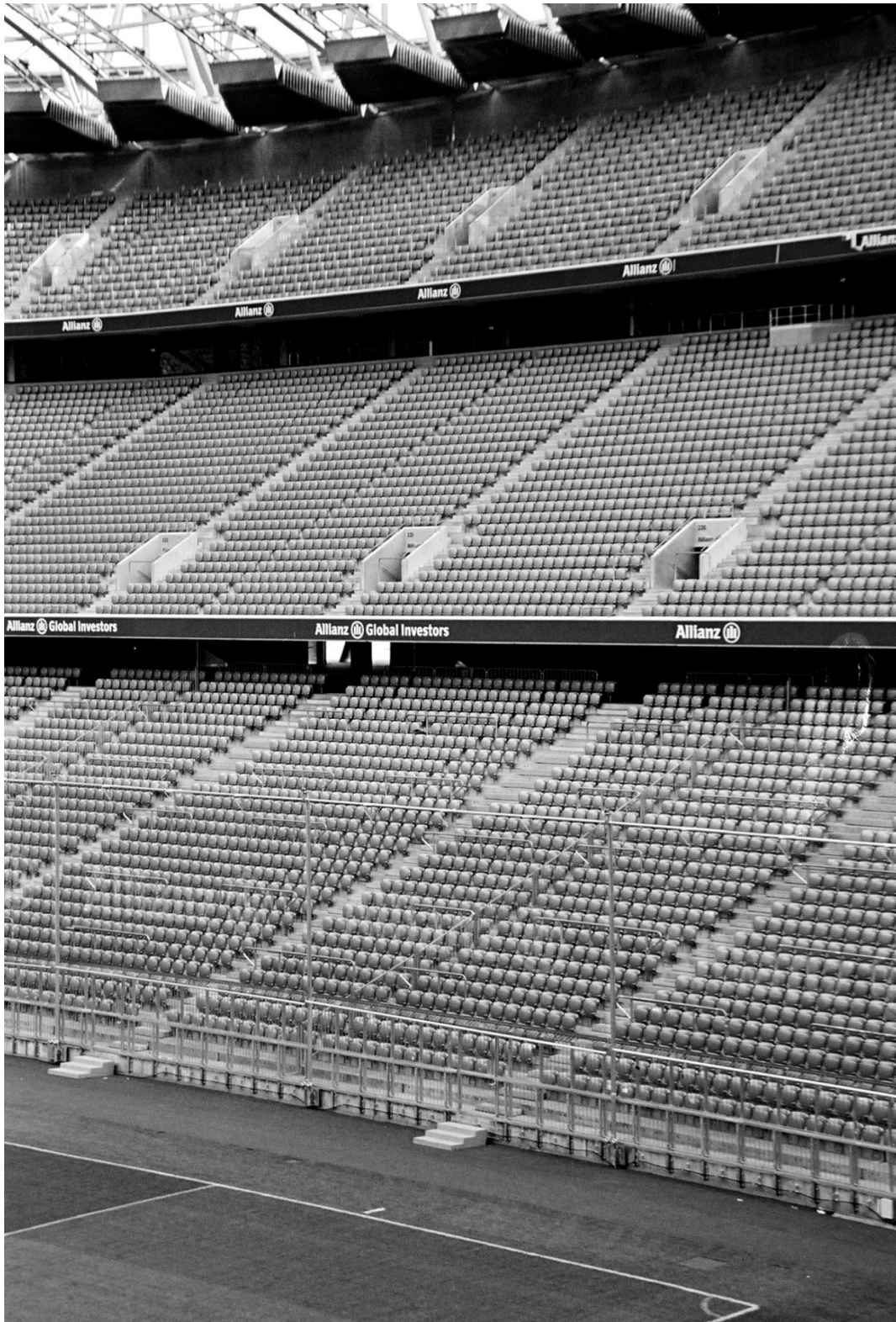
Figure 3. Allianz Arena, Munich (2006) - example of three-storey stands with a rectilinear profile. The slope of the third floor is 35°. The elevation of the last row of seats reaches a value of about 40m. (Photo: M. Pelczarski)
