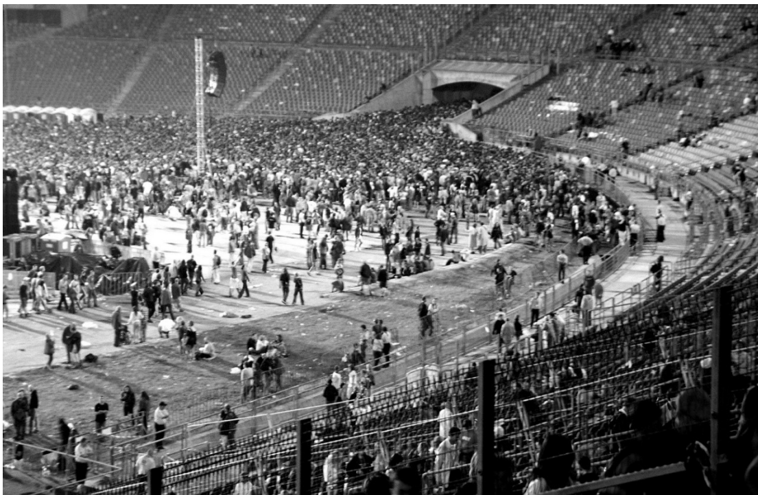
Figure 7. The Silesian Stadion, Chorzow, Poland - fragment of the arena in the area of the southern tunnel. Sustainable Infrastructure (2018)
