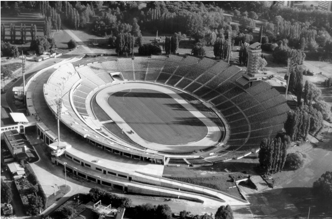
Figure 1. The Silesian Stadion, Chorzow, Poland - aerial view from the north, the state in 2006. On the left side seen ramps serving eastern sectors, under which there is a room complex of total floor area of 18,000 sqm; stadion capacity: 47,000 seats for spectators. (Photo: T. Najdzien, 2006)
