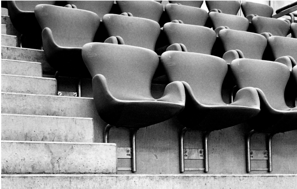
Figure 4. Allianz Arena , Munich (2006) - example of the relationship between the geometry of the stairs and stand steps; each stand step corresponds with three stairs steps. (Photo: M. Pelczarski)
