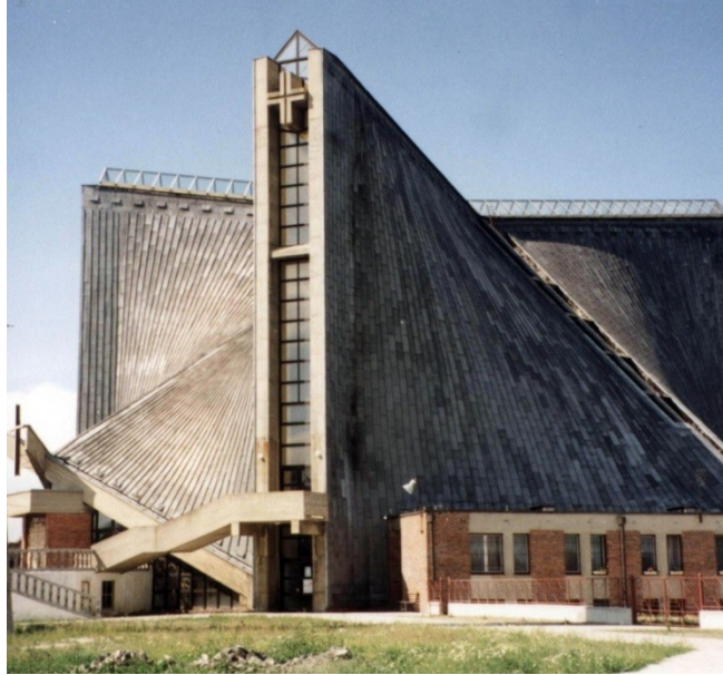
Figure 5a). W. Kurowski, W. Marszalek at alt. – St. Joseph the Worker church in Zgorzelec, Poland, 1983: general view on multi-hyper concrete roofing (Marszałek at alt, 2012)
