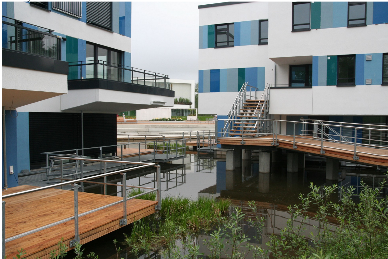
Figure 2. Wilhelmsburg, Hamburg - the Waterhouses on piles in the middle of an exhibition area. Photo by the author.
