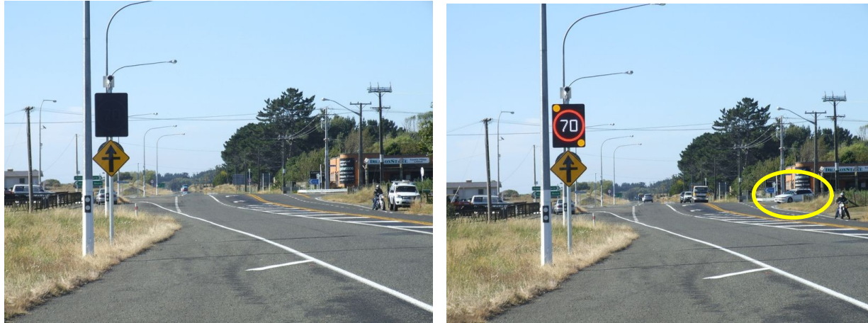
Figure 2. The RIAWS in operation at Himitangi with no conflict risk (left) and a potential conflict risk (right) with a side road vehicle present (circled).
