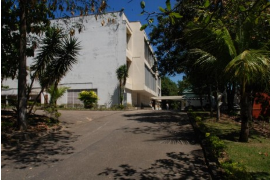
Figure 6a - Building on the IEN installation.
