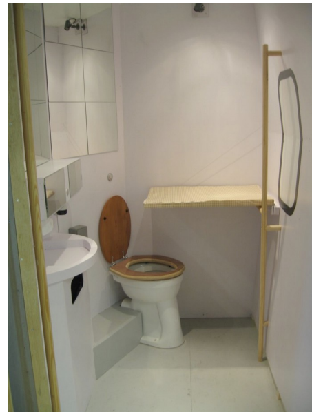
Figure 2. Interior of Family sit toilet
