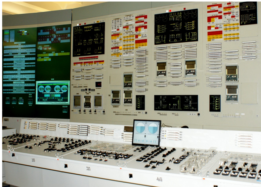
Figure 3. Ecological display in the FSS (LCD VDU with resolution of 1280×1024 pixels and screen size of 300 375 mm is used)
