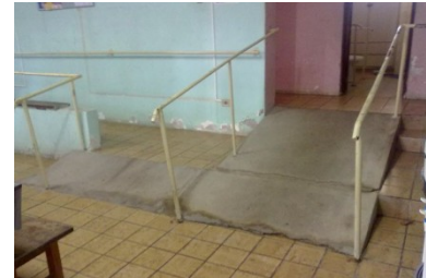
Figure 3. Existing ramp in ILPI 2. (Authors, 2012)
