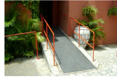
Figure 6. Existing ramp in ILPI 2. (Authors, 2012)
