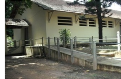
Figure 12. Existing ramp in ILPI 4. (Authors, 2012)
