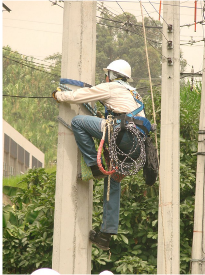
Figure 1. Climbing to utility post
