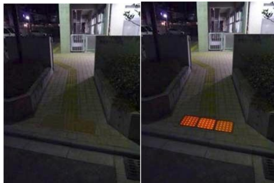
Figure 3. Nighttime visibility of studded paving blocks (left: conventional blocks, right: blocks under development)
