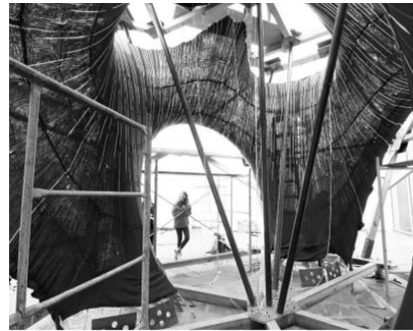
Figure 4 and 5. Knit Candela Pavilion. A concrete waffle shell built using a lightweight, stay-in-place, cable-net and knitted fabric formwork.
