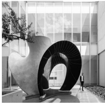
Figure 4 and 5. Knit Candela Pavilion. A concrete waffle shell built using a lightweight, stay-in-place, cable-net and knitted fabric formwork.
