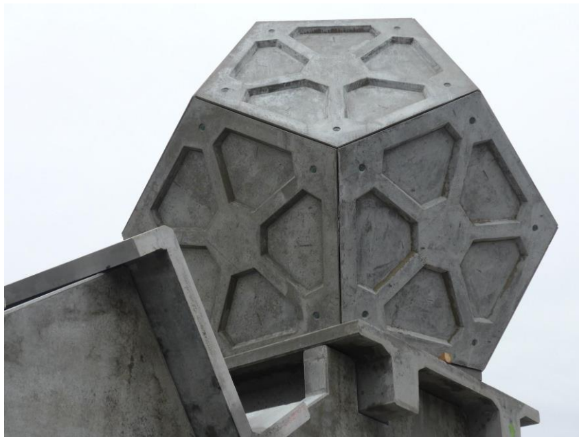
Figure 1. The panel structure composed of thin-walled concrete slabs
