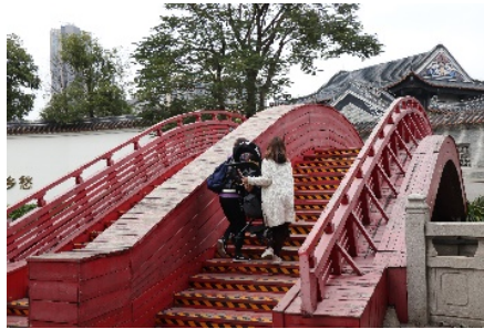
Figure 4: Arched wooden bridge with poor accessibility.
