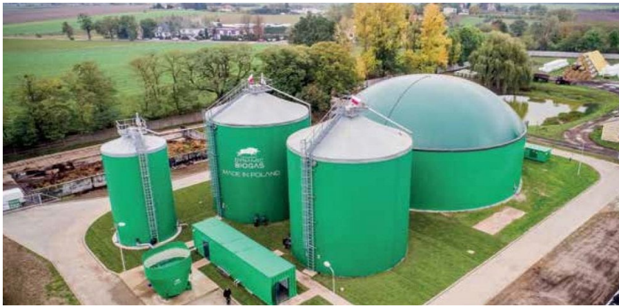
Figure 4: Domains of biogas plant (CHP) farm from greater Poland region.
