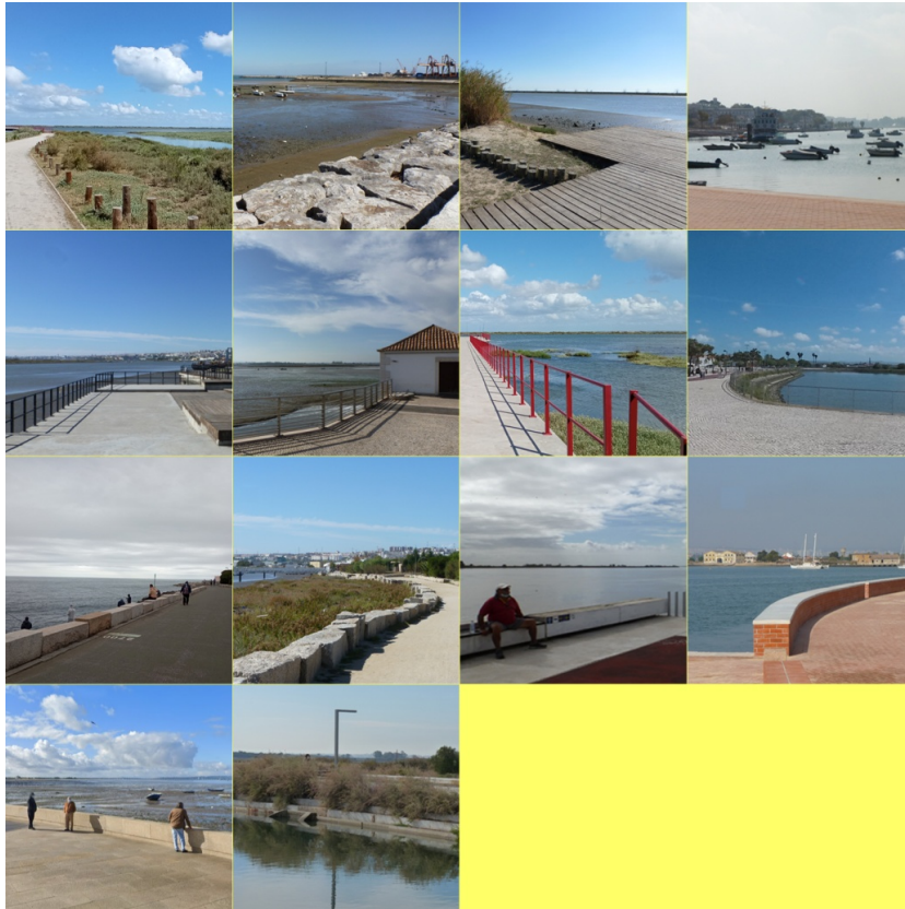
Figure 1: Different kinds of water limits: from a complete absence of physical protections – promenades elevated above the flood area or ground sloping towards the water (top) – to barriers that are high but as transparent as possible, to low opaque walls, and a few high opaque protections (bottom). (Author’s photographs).
