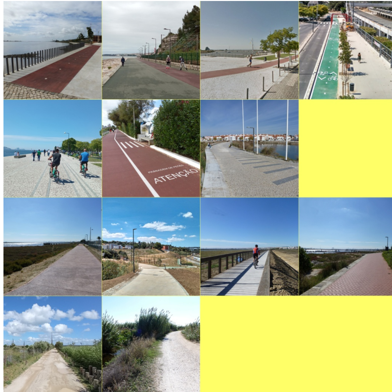
Figure 2: Different kinds of cycling/pedestrian paths: from uniform promenades (bottom) – with a minimum of elements added to often pre-existing maintenance paths – to subtle elements in the pavement that mark paths for ‘soft mobility’, to the presence of a preferential lane highlighted by bright colours (top). (Author’s photographs).
