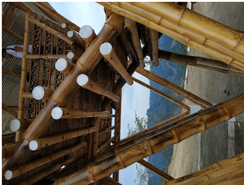
Figure 3: Bamboo structure built by the INBAR team.
