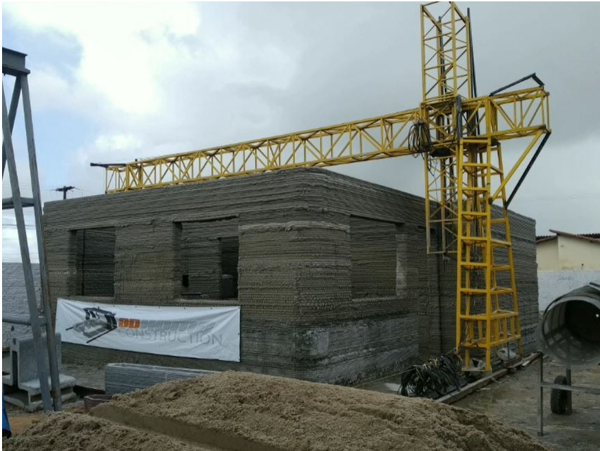
Figure 2: Prototype housing structure inspired by the wikihouse. Source: Nardeli; Pereira, 2017.
