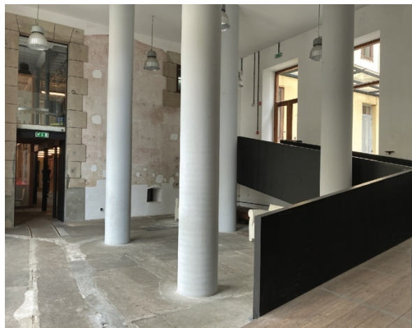
Figure 3: FCCVA's interior space. (Gaëlle Pillault, 2020).
