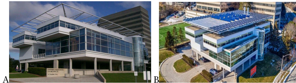
Figure 1: OAA building before (A) and after (B) the renovation.
