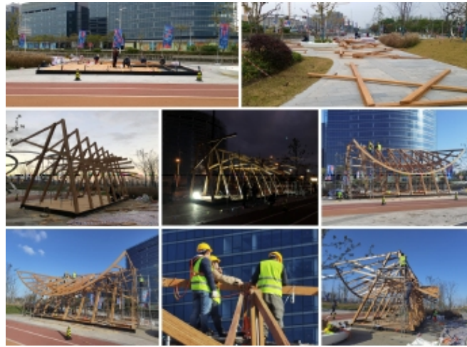
Figure 1: On-site installation of factory prefabricated assembled components (Author's own photos).
