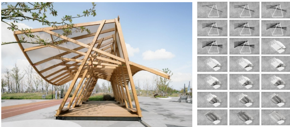
Figure 5: Triangular structure of the post (Author’s own photo).
