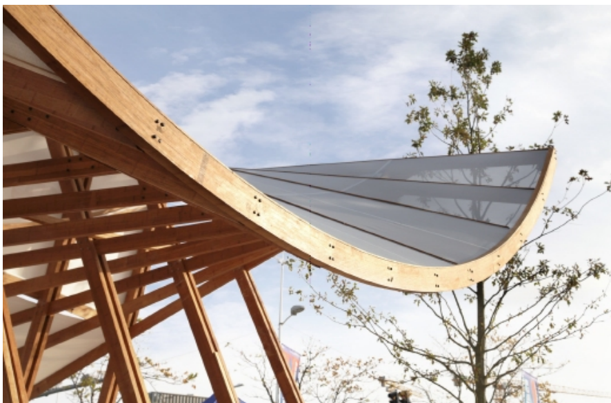
Figure 6: The wooden spokes rotate around the bearings while translating, solidifying the trajectory of the bicycle wheel. (Author’s own photo).
