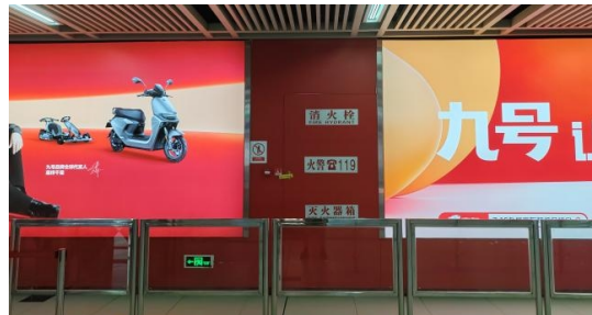
Figure 13: The advertising wall in the subway is affecting the fire hydrants (Wenyi Xu, 2023).
