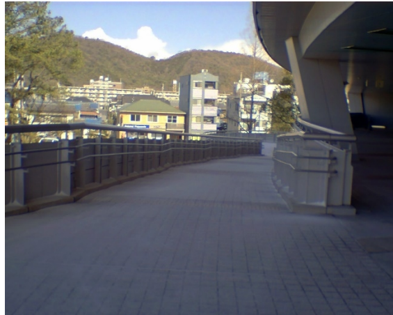
Figure 7: Gentle slope going downward, the Okayama Stadium.
