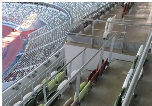
Figure 3: Sight line is secured: two front rows are removed, the New National Stadium.
