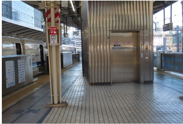
Figure 10: Original elevator reserved for staff in Tokyo Station. It has existed for more than 25 years, and passengers who use wheelchairs were cordially invited to use this.
