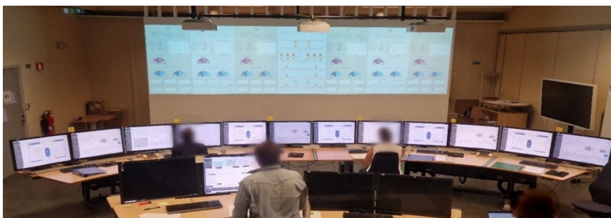
Figure 3: Ongoing tests in the HSMR simulator with a two-person crew (a process expert is behind).
