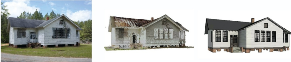
Figure 2: Progression of creating precision specification of Tankersley school using standard photography (left) and LiDAR point cloud technology (center) to create a precision BIM model (right) (image provided by author).
