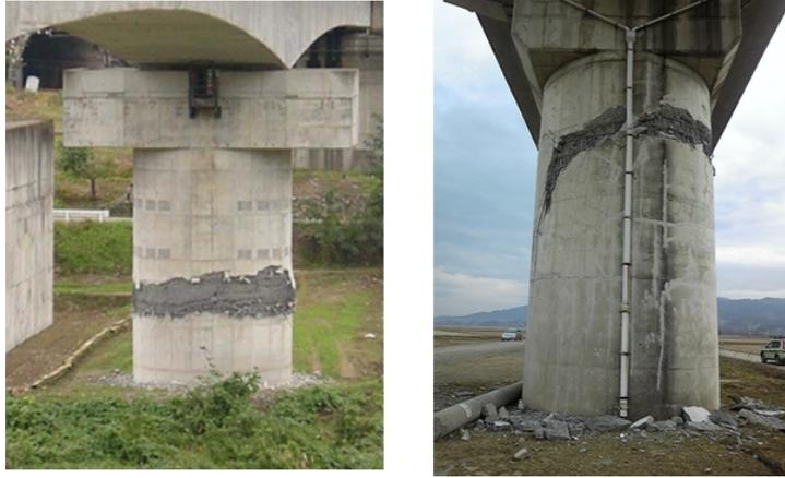
**Figure 1:** Damage to RC piers after earthquake.
