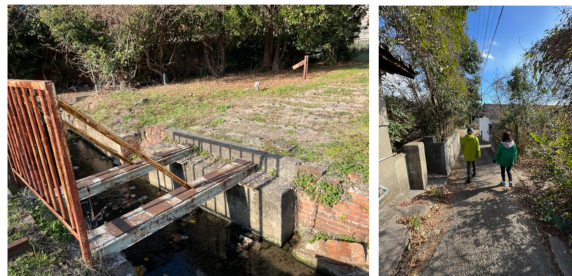
Figure 4: Risk checks by walking on-site.
