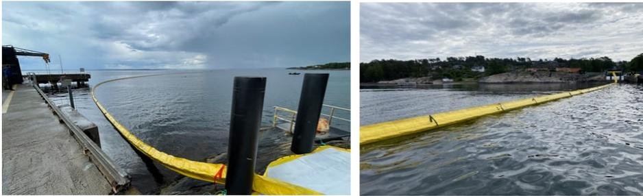
**Figure 1:** Inflatable dams to limit the expansion of the oil bed.
