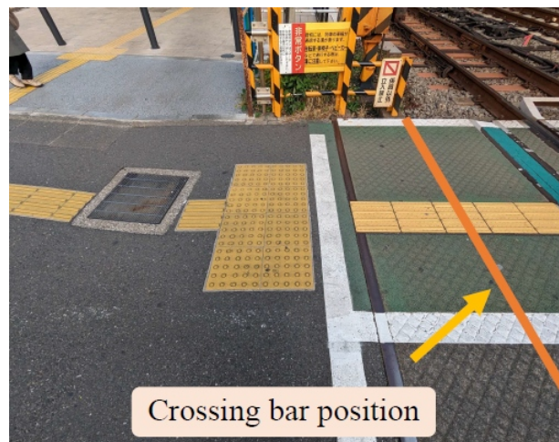
Figure 7: Condition of the railroad crossing boundary (north side of the crossing).
