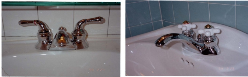
Figure 7: & 8: Water sink faucet with two levers to activate hot- and cold-water flow, and cross-type handles to do the same. The right one is a replaced version of the left example. Therefore, one has to turn right to activate cold-water flow although the design suggests the opposite (photos by author).
