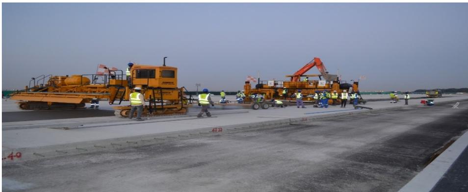
**Figure 1:** Paving of apron with slipform paver.
