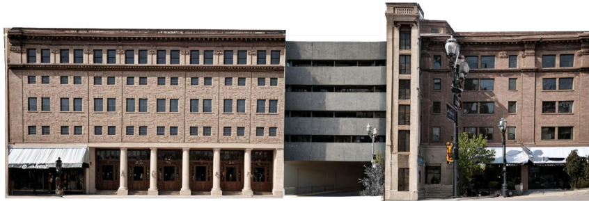
Figure 6: Final picture of building with material and colors.
