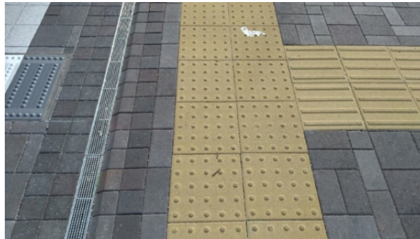
Figure 2: Example of tactile walking surface indicators installed at a pedestrian crossing.
