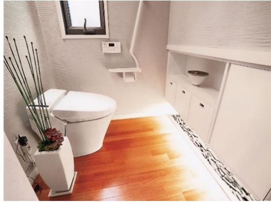
Figure 9: Toilet diagonal handrail.
