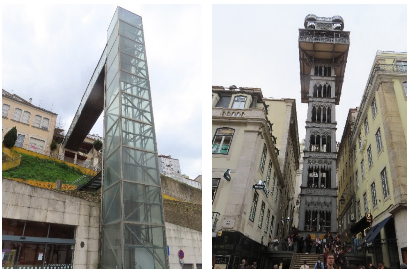
Figure 7 & 8: Elevators, Coimbra and Lisbon, Portugal.
