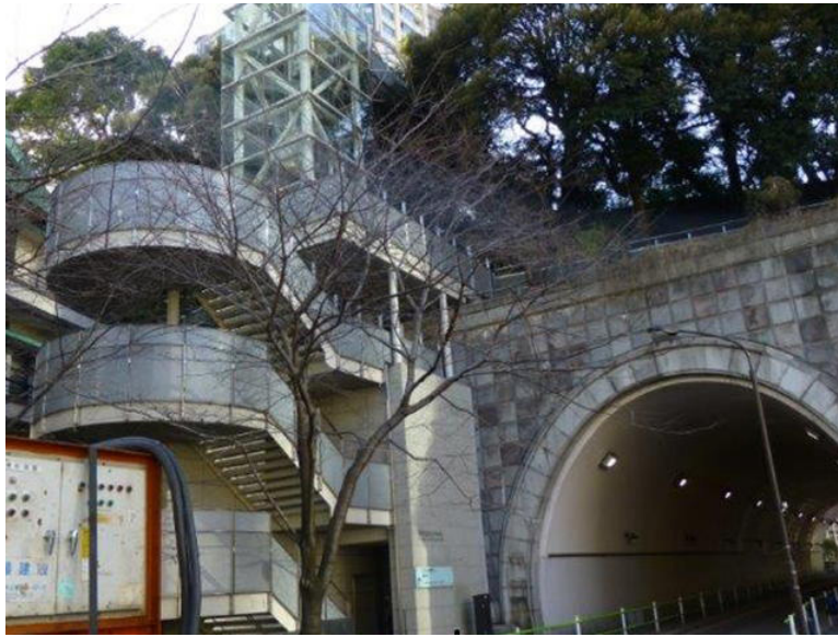
Figure 9: Elevator, Atago, Tokyo, Japan.
