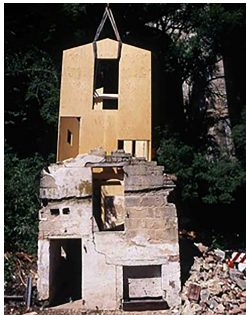
Figure 2: S(ch)austall project assembly sequence. Source: https://maderayconstruccion.com/un-corazon-de-madera-schaustall-en-eiswoog/ (Access: November 27, 2025).
