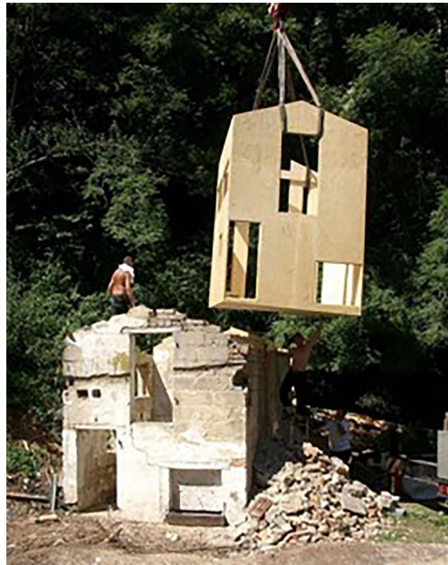
Figure 1: S(ch)austall project assembly sequence. Source: https://maderayconstruccion.com/un-corazon-de-madera-schaustall-en-eiswoog/ (Access: November 27, 2025).
