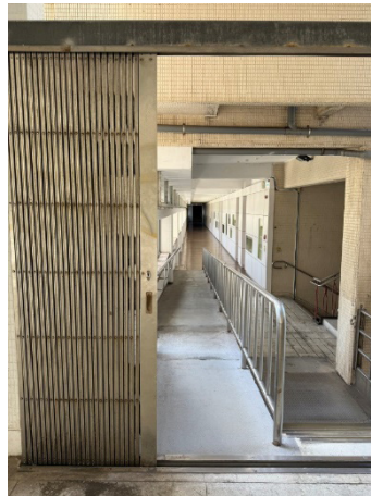
Figure 3: Current state of the ramp entrance.
